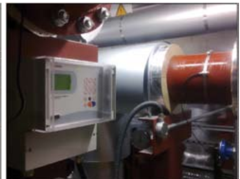
Aysix 150 for heat quantity measurement application using PT100 sensors
